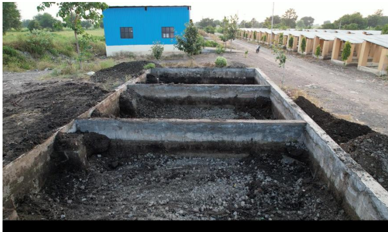
Upgradation from Unplanted Drying Bed (UPDB) to Planted Drying Bed (PDB)
