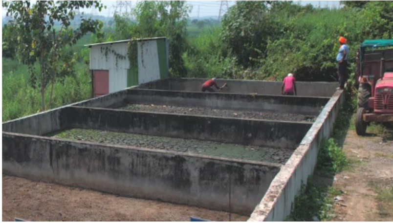
Upgradation from Unplanted Drying Bed (UPDB) to Planted Drying Bed (PDB)
