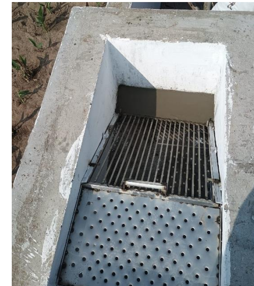
Addition of Screen Chamber at receiving station
