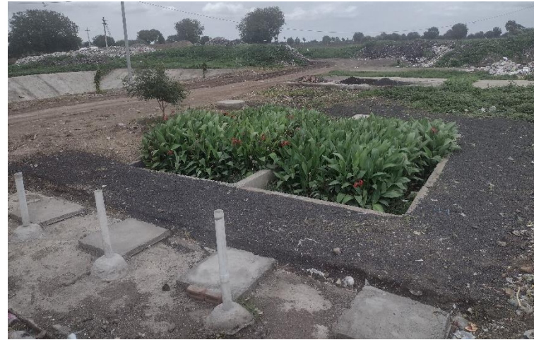
Filter media replacement at Planted Gravel Filter
