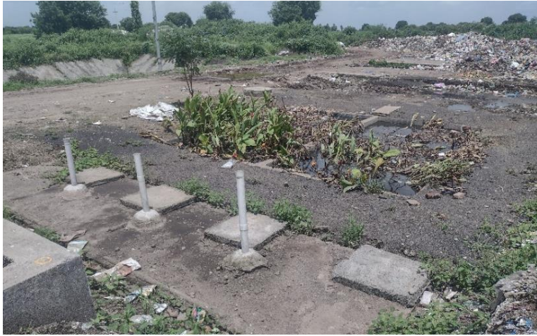
Filter media replacement at Planted Gravel Filter
