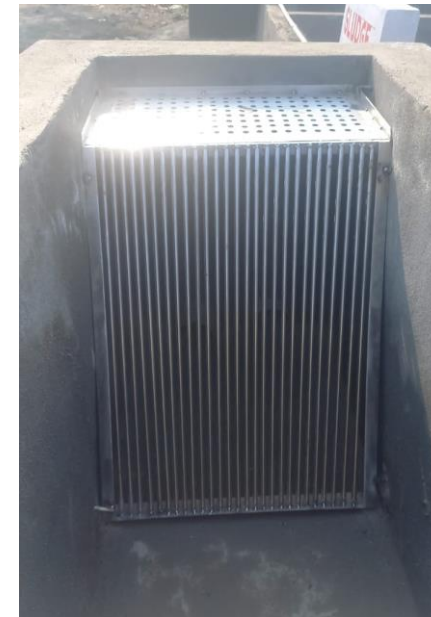
Addition of Screen Chamber at receiving station
