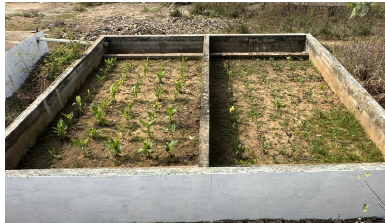
Filter media replacement at Planted Gravel Filter
