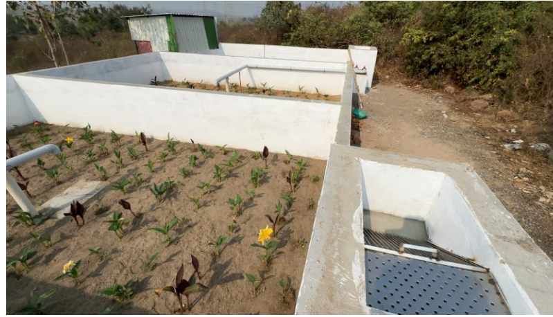
Upgradation from Unplanted Drying Bed (UPDB) to Planted Drying Bed (PDB)
